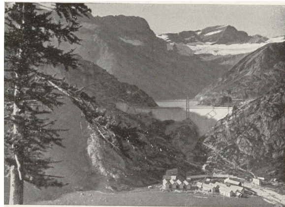
Waterpower plant build in Barberine in 1923 owned by the Swiss Federal Railways with an electricity production of up to 15000kW and an embankment dam capacity of 39000000m 3 .
